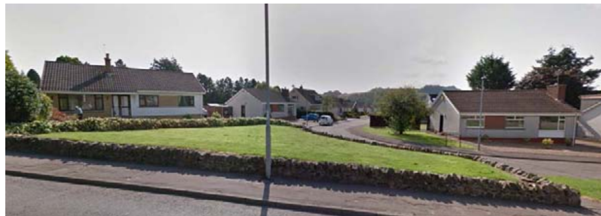
One storey high predominantly brick and render at Dollar Road in a variety of architectural styles (looking South)
