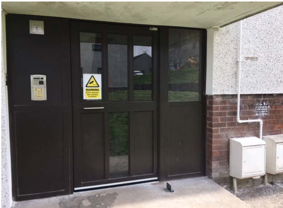
Secure Door Entry Upgrade – Branshill Park Sauchie
