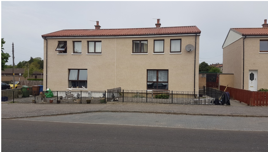
Non-Traditionally Built Upgrade – Clackmannan Lochies Road
