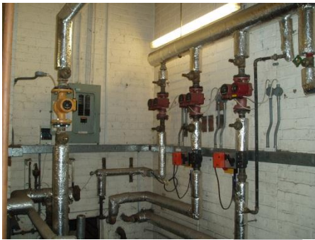
Plant room heating pipework is generally in good condition but requires some modernisation and replacement insulation.
