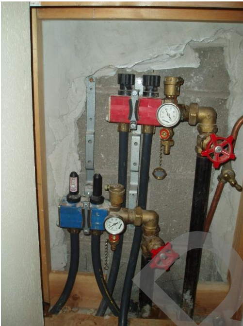
Underfloor heating manifold to Meeting Room
