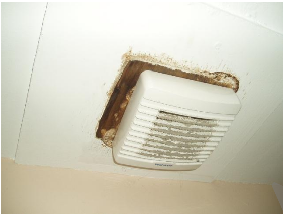
Vent Axia toilet extract fans in poor condition.
