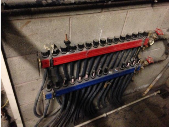
Underfloor heating manifold to Sports Hall
