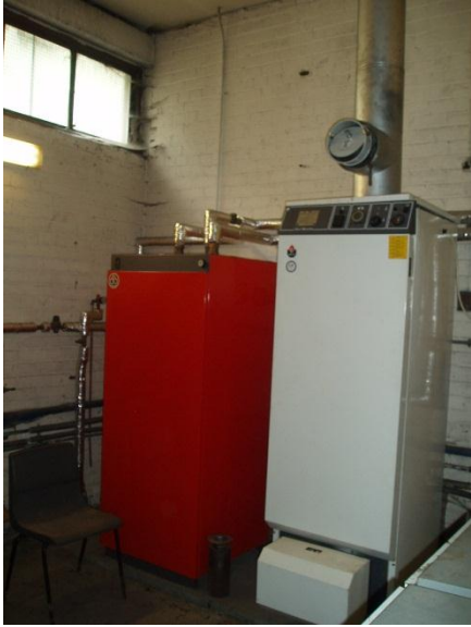
1No ACV Heatmaster gas fired hot water boiler linked to 1No ACV storage vessel.
