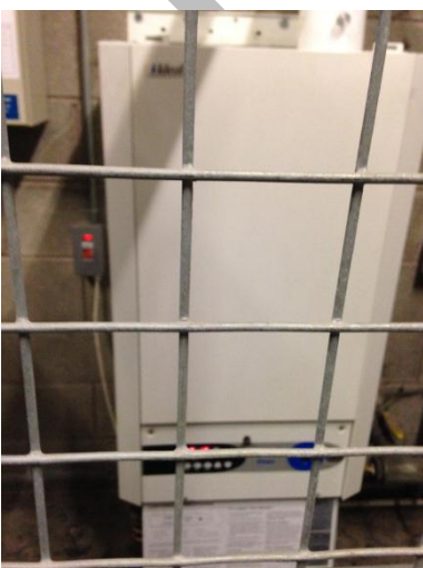
1 No Ideal Imax gas fired atmospheric boiler installed in Meeting Room overlooking Sports Hall. This boiler serves underfloor heating manifolds to Sports Hall and Meeting Room. Visually the unit is in good condition.
