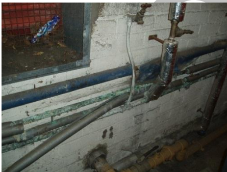
Cold water mains pipework in very poor condition showing signs of major corrosion and lacking sufficient insulation.
