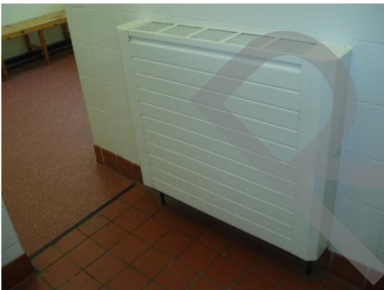
LST radiators installed in circulation areas are in good condition.
