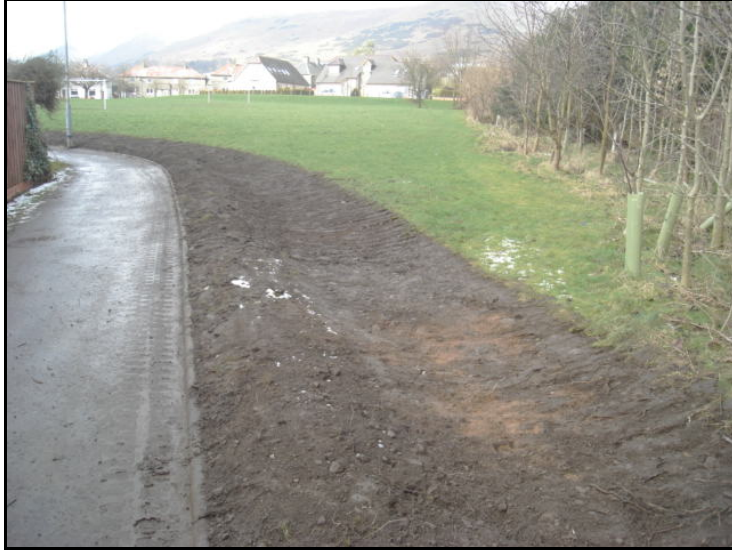
Completed swale to capture flows at Drum Court, Dollar - 06/03/09
