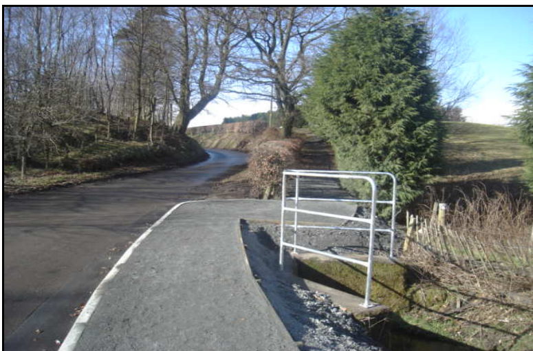
Back Burn Culvert at Muckhart Golf Club - 09/03/09
