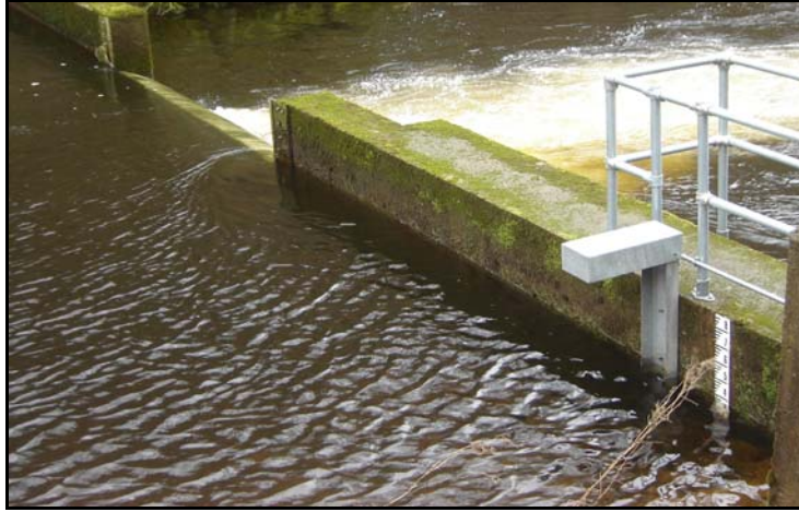
Flow / level gauging station at the river outflow from Castlehill Reservoir - 16/03/09
