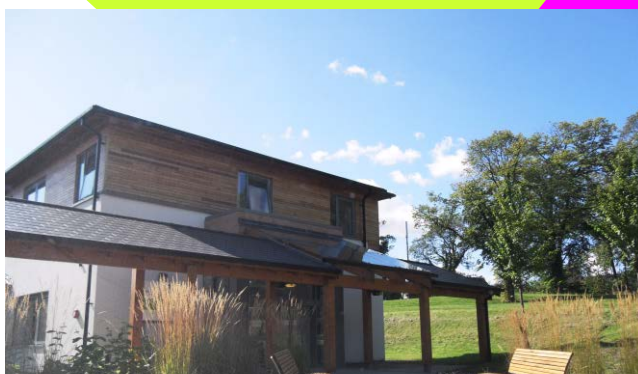
The Mental Health Resource Centre is a purpose-built building which accommodates our Day Unit service and Community Mental Health Team as well as Consultant Psychiatrists, Psychologists and Art Therapy who we work jointly with to provide our services.
