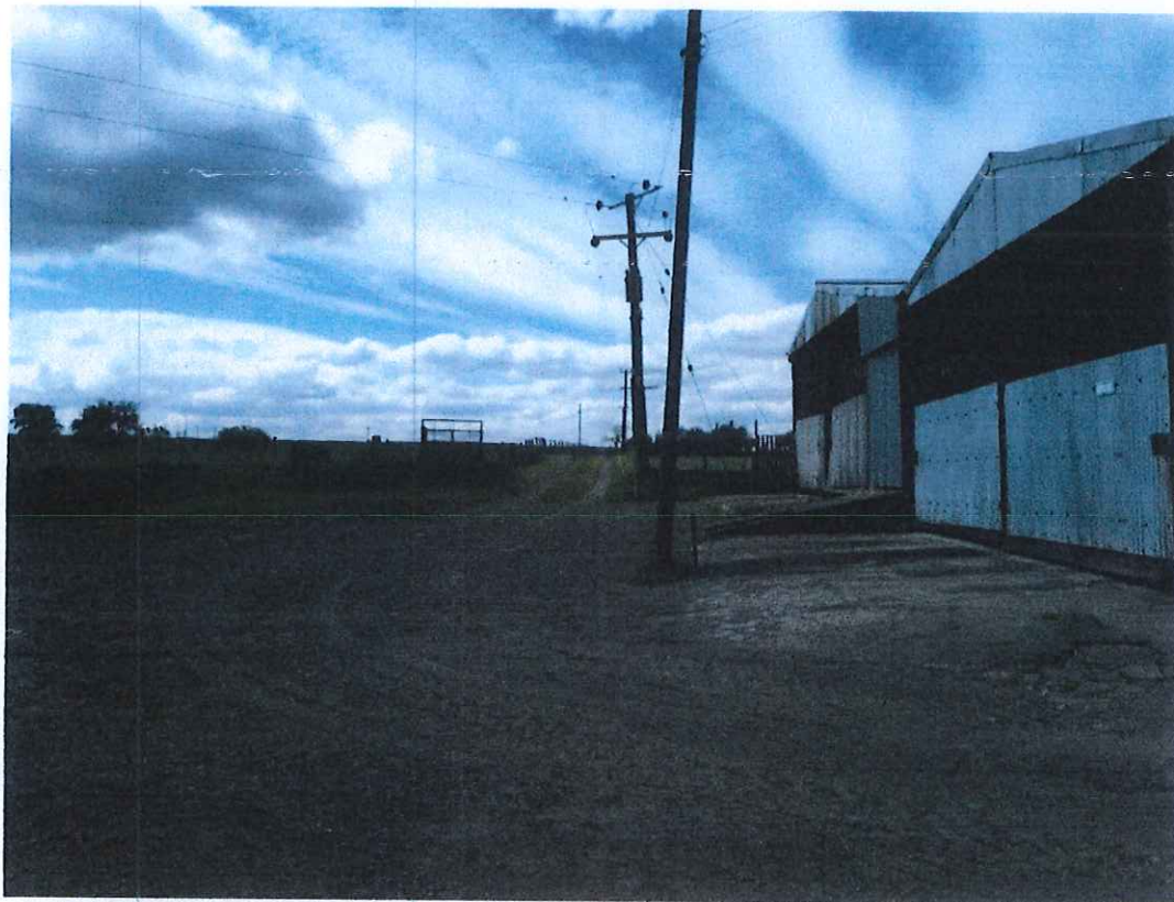
Existing Barns and new access road
