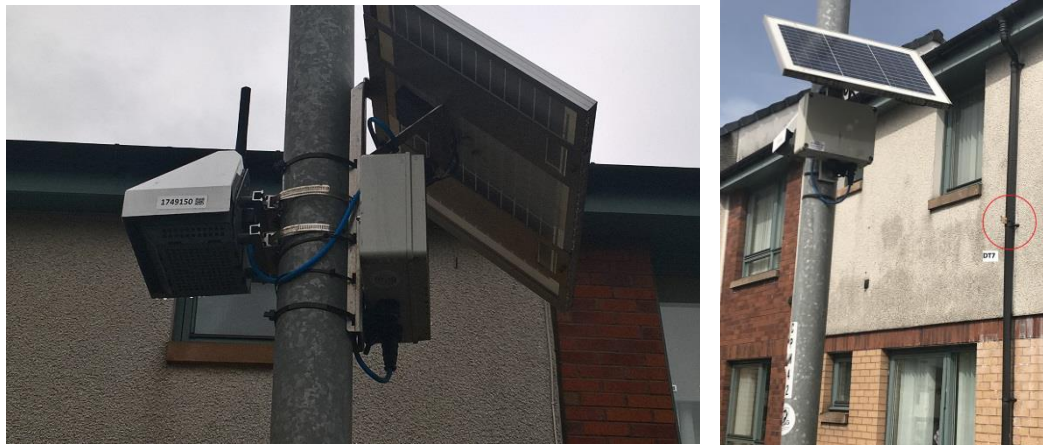
Figure 3.2 – AQ Mesh Unit and DT7 on Location at Hallpark Road, Alloa
