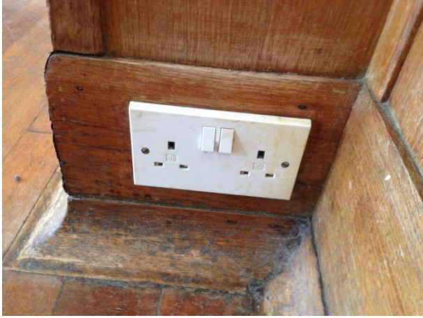
Socket within the wooden skirting
