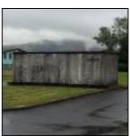
Rotting timber louvered plant room doors identified for replacement.
