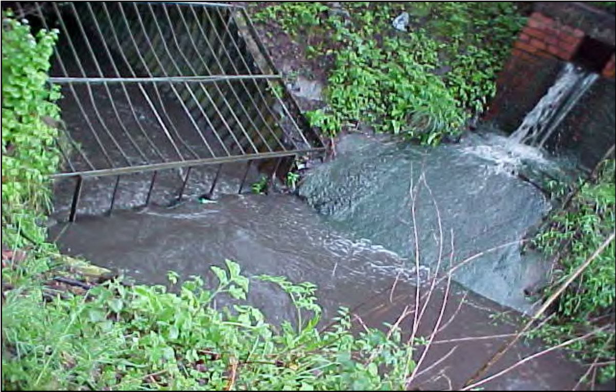
Photo 4 - Brothie Burn at Shillinghill Culvert, Alloa – 10/05/04
