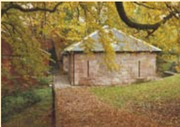
Old pump house
