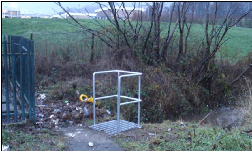
Photo 11 - New Trash screen, handrail and access footpath at Ormiston Drive, Alloa – 12/12/06
