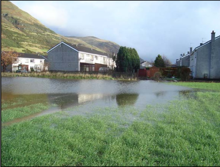
Photo 7 - Overland flow affecting Cleuch Drive, Alva – 20/11/06
