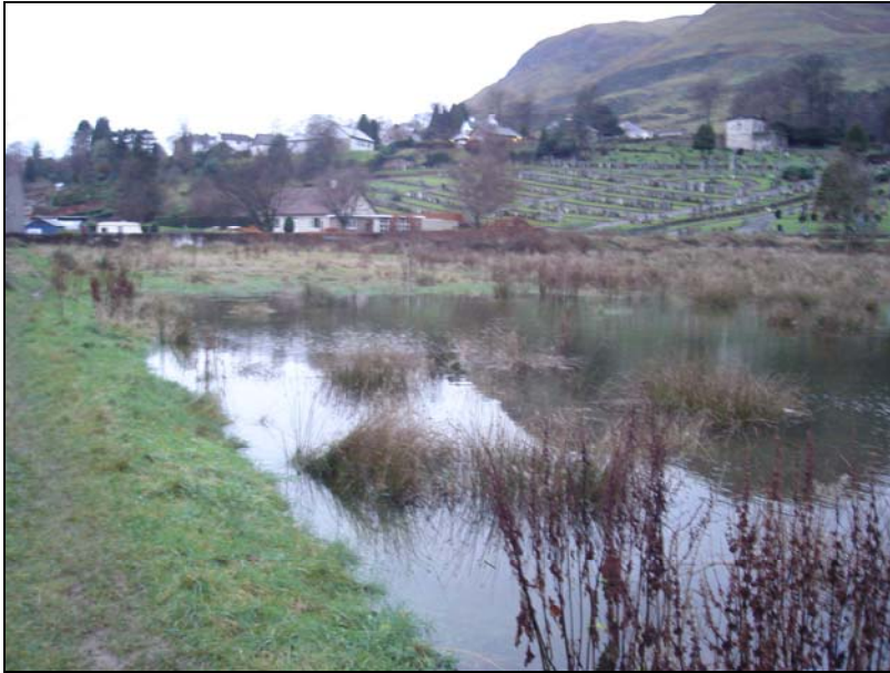
Photo 6 - Flooding to north of Properties at 41 to 55 Rhodders Grove, Alva – 14/12/06
