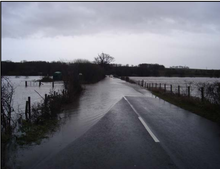
Photo 8 - B908 inundated by River Devon floodplain – 14/12/06
