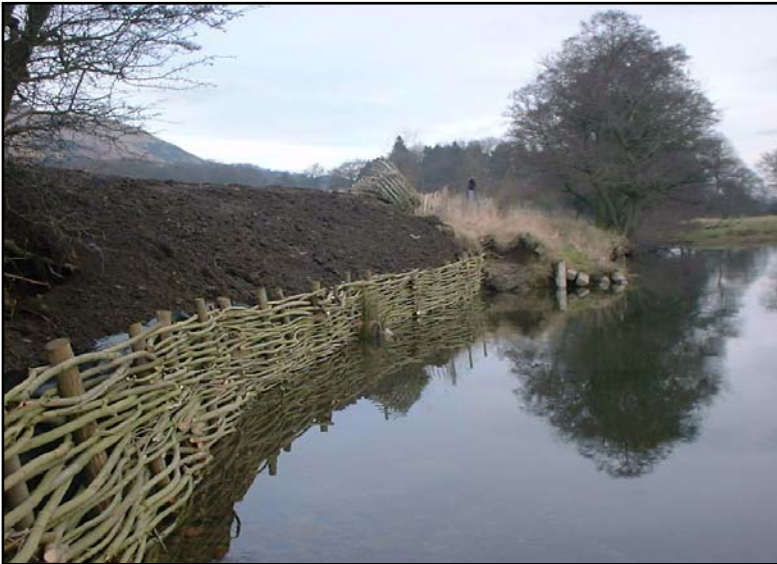
Photo 22 – Willow walling of the north bank of the River Devon between Tillicoultry and Dollar
