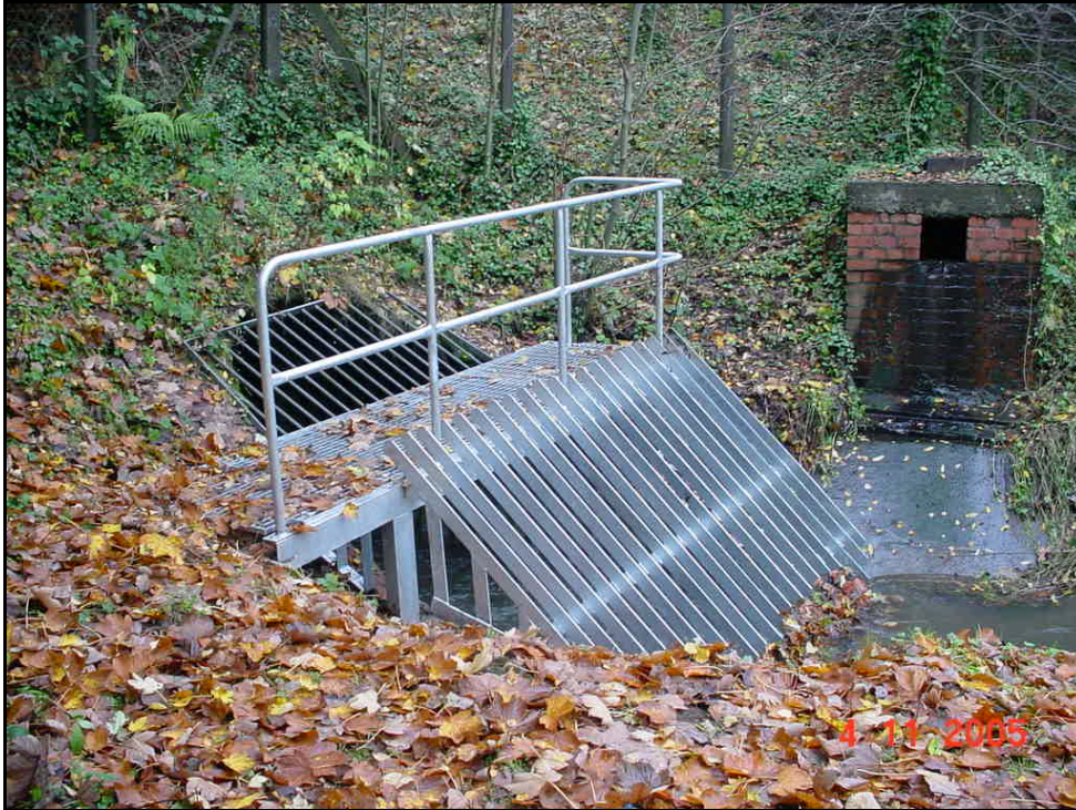
Photo 4– Brothie Burn Trash Screen at Shillinghill Culvert, Alloa
